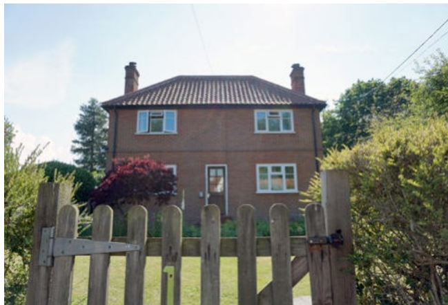
Interwar detached house west of King Street but not included within the Conservation Area boundary
