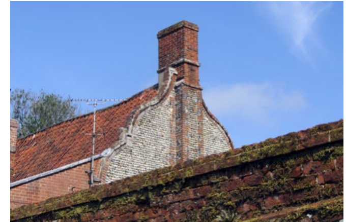
Shaped gable of Hunworth Hall from Stody Road
