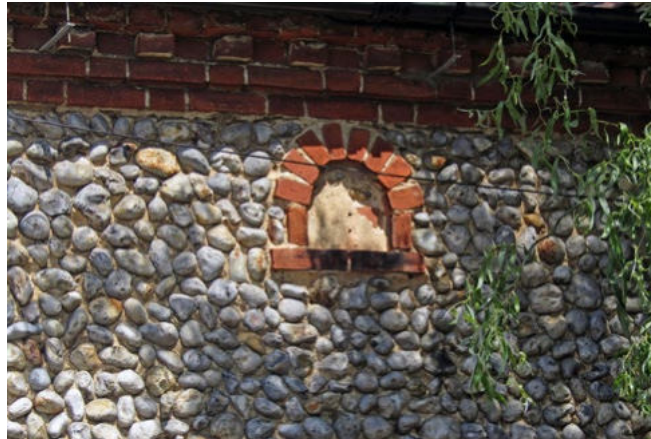
Detail of brick and flint decorative embellishment on cottage wall
