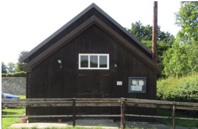
Close view of the front elevation of the Village Hall
