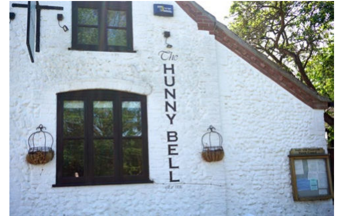
Detail of windows and painted lettering facing the Green
