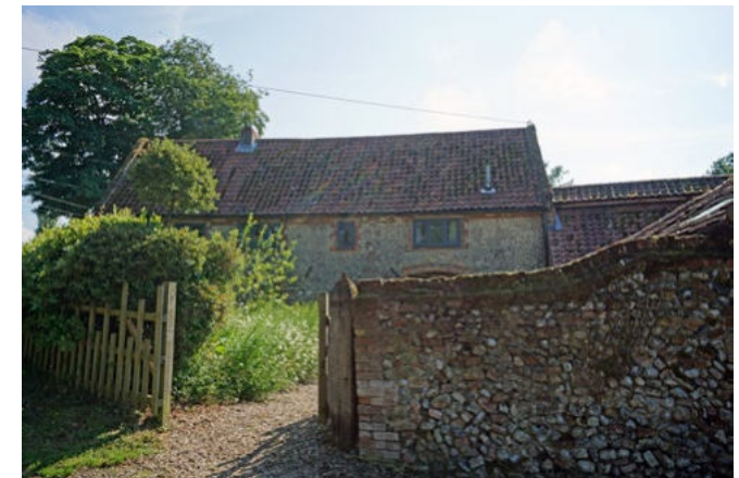
Converted barn at Hunworth Hall Farm
