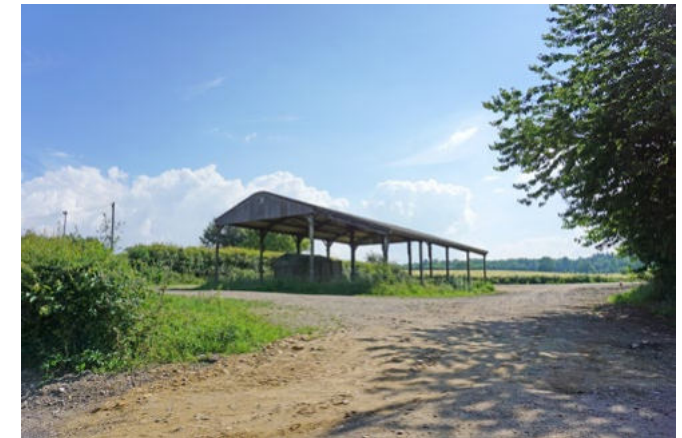
Modern agricultural barn seen from King Street
