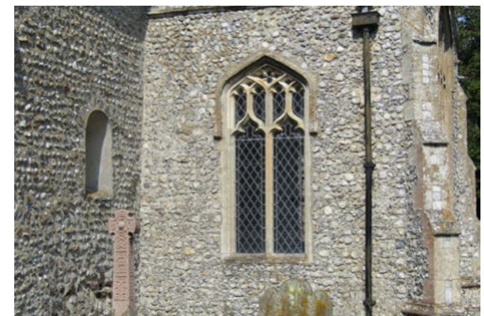
Detail from south elevation of the church showing two phases of windows
