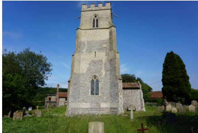
The west tower showing the embattled parapet roof
