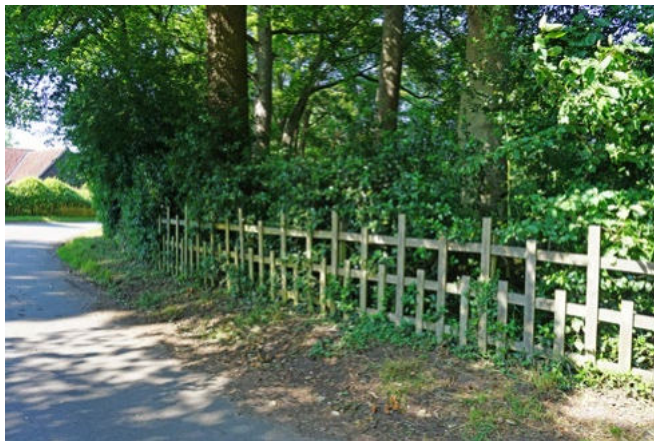
Fence at the Study Road/King Street junction
