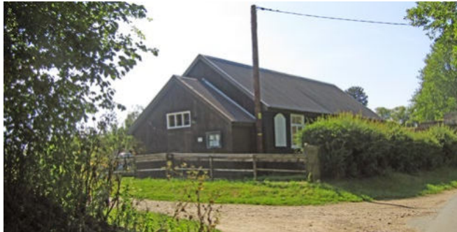
View of the Village Hall from King Street
